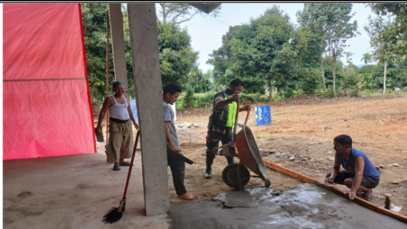
Gambar. 1 Proses Renovasi Lantai Balai Baca
